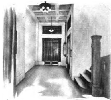
Entrance to Public Elevators
